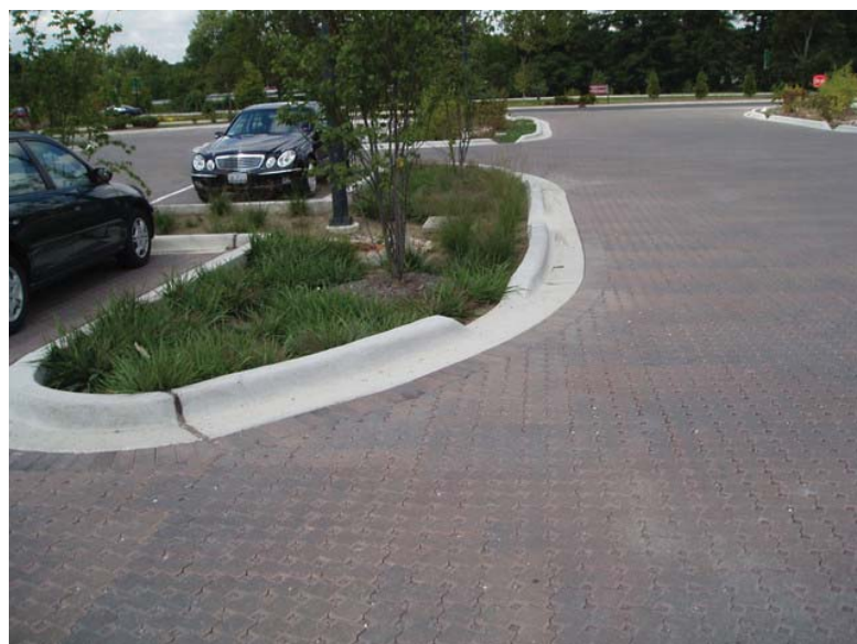
Permeable pavers combined with recessed planted islands slow surface runoff in parking lot areas.
